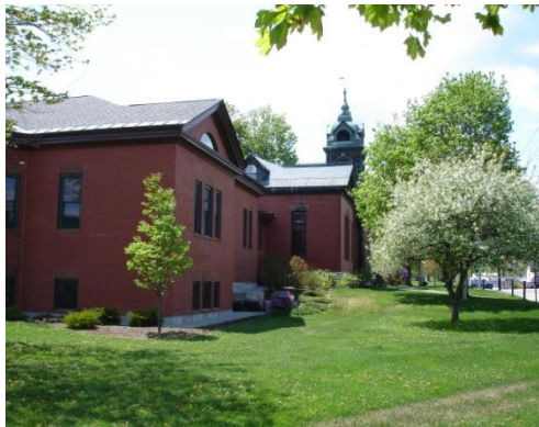
Conway Public Library, facing east, with the addition in the foreground
